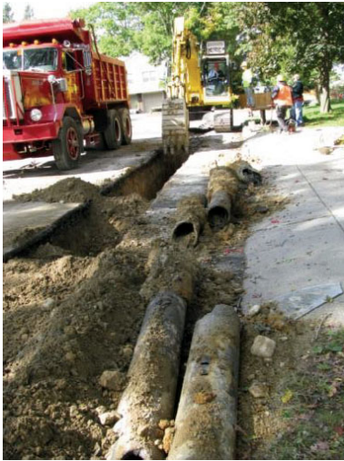
Water Main Replacement Construction
