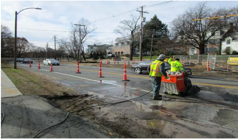
Lane Restriction and Traffic Control on Commonwealth Avenue
