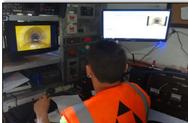
Sewer TV Inspection
