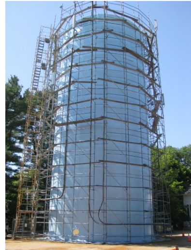
Rehabilitated Water Storage Tank
