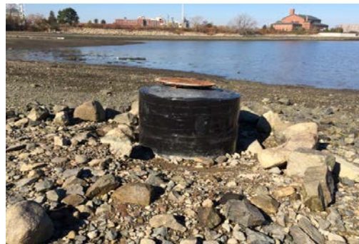
Sewer Manhole at Beach - Raised and Sealed
