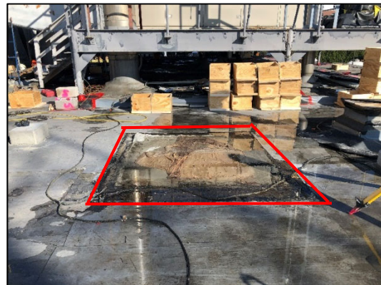
Typical Roof Infill for Abandoned Exhaust
